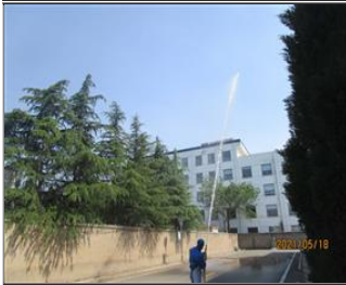
Photo of fire safety equipment Firefighting facility test.JPG
