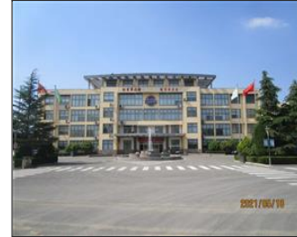
External photo(s) of the production unit(s) Office building.JPG
