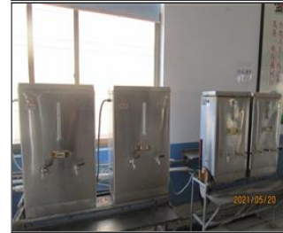
Photo of the sanitary facilities Drinking water.JPG
